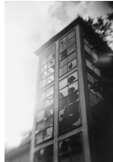
Broken windows. Pilot Training Camp in Jüterbog
