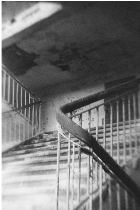
Staircase. Pilot Training Camp in Jüterbog
